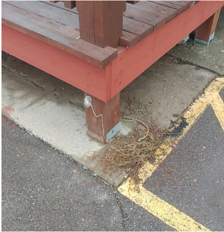
The footings and piers are in Satisfactory Condition.
