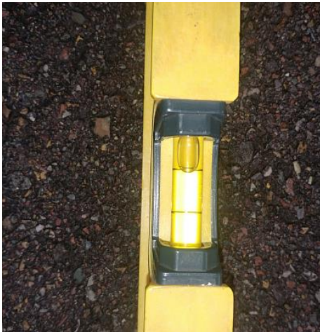
The driveway is properly pitched away from the building.
