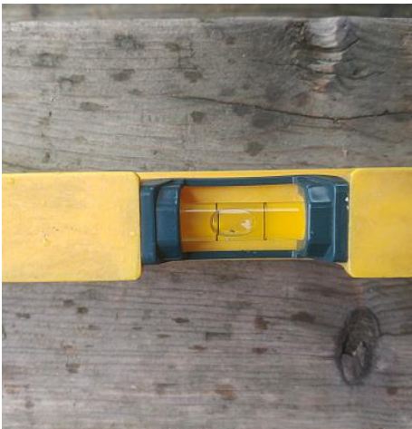
The steps are properly pitched.
