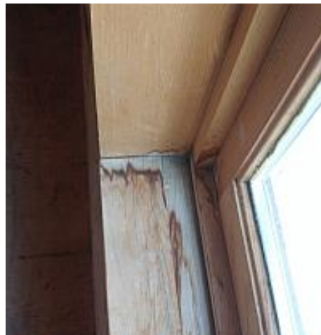
Moisture stains observed on the window sill. Although the area tested dry with a moisture meter, the stains came from somewhere. Recommend Repair.
