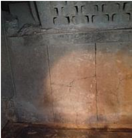
The cracked fire bricks are typical. The door gasket is showing expected indications of wear.
