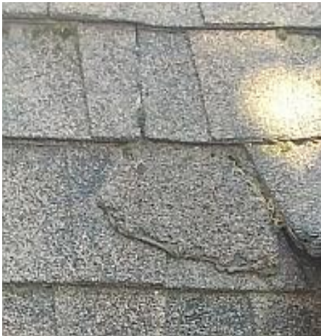
Broken/missing shingles observed. Granule loss observed. Recommend Repair/Replacement.
