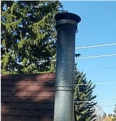
Indications of creosote buildup observed. Recommend cleaning and seasonal cleaning thereafter.
