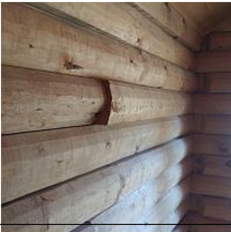
Numerous offset logs observed. This home is constructed of single tongue and groove milled logs. These types of log are designed to fit tightly together. The tongue and groove should help minimize the type of offsetting observed.
