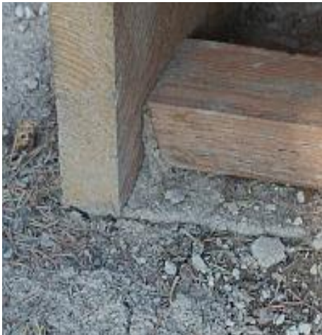
Proper treated wood used for contact with concrete.
