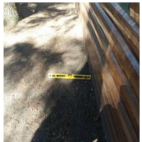
Negative grade observed in several areas. Recommend Repair (backfill).
