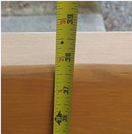
The railing is the proper height.
