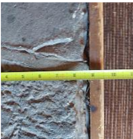
According to the owner’s manual there should be 16 inches of hearth in front of the unit. The hearth only extends 9 inches to the front of the unit. This is a potential Safety Hazard. Recommend Repair.
