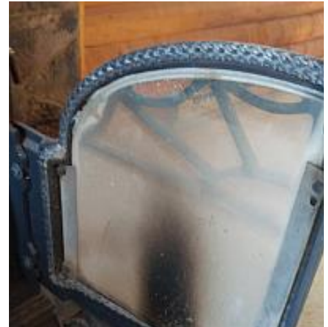
The cracked fire bricks are typical. The door gasket is showing expected indications of wear.
