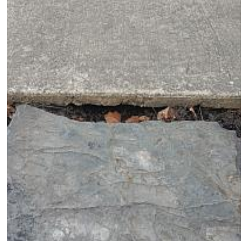
Material has eroded from underneath the service walks. Recommend Repair (backfill).
