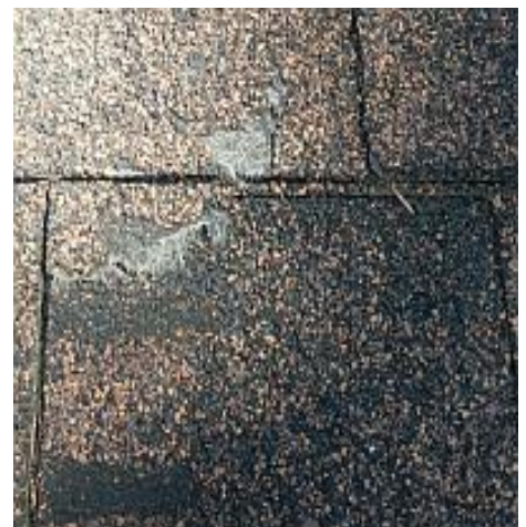
Broken/missing shingles observed. Granule loss observed. Recommend Repair/Replacement.
