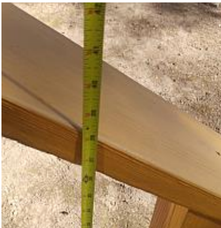
The railing is the proper height.
