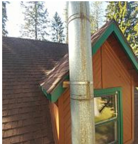
Indications of creosote buildup observed. Recommend cleaning and seasonal cleaning thereafter.
