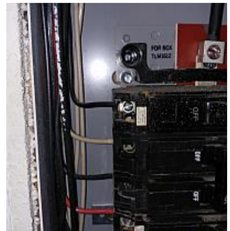
White (neutral) wires used as black (live or line) wires should be color coded black.
