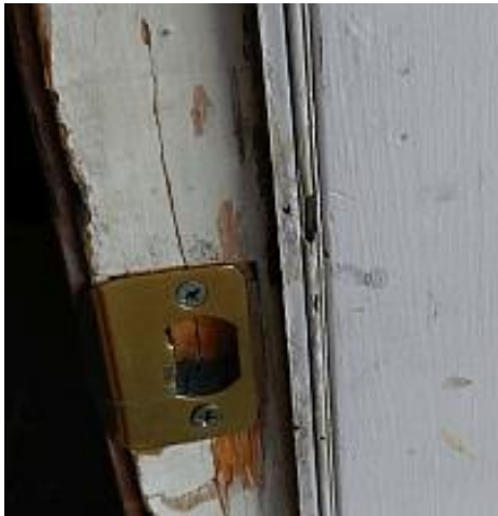
The weather stripping is torn/holed. The door frame is cracked. Recommend Repair/Replacement.
