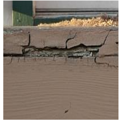
The floor is deteriorated in several areas. This is a potential Safety Hazard. Recommend Repair/ Replacement.
