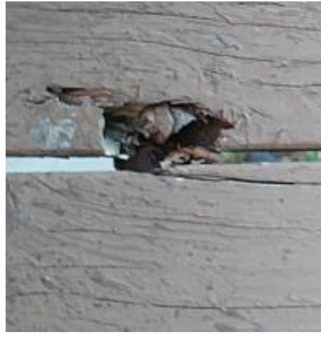
The floor is deteriorated in several areas. This is a potential Safety Hazard. Recommend Repair/ Replacement.
