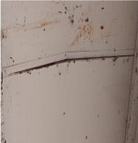
The soffit is loose in several areas. Recommend Repair.
