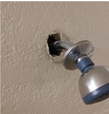
Recommend calking where indicated to help prevent moisture penetration into the walls.
