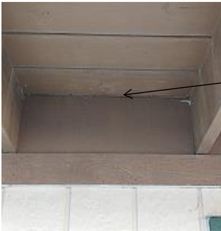
The floor is not flashed. Flashing helps prevent moisture intrusion at the deck/home junction. If the floor is ever replaced recommend flashing be added.
