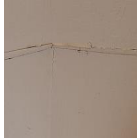
The soffit is loose in several areas. Recommend Repair.
