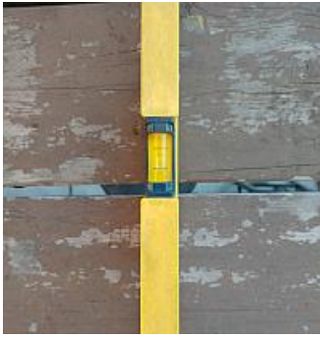
The floor is properly pitched away from the home.
