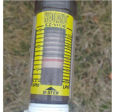
The flow rate is 14gpm, which is within acceptable limits.
