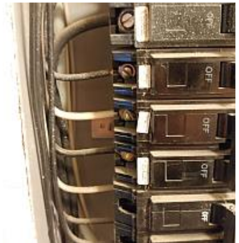
White (neutral) wires used as black (live or line) wires should be color coded black.
