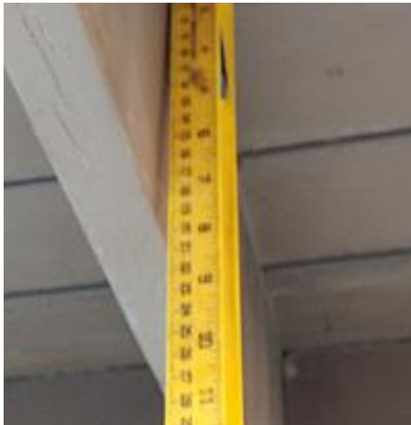
The floor is cantilevered 47 inches. According to current standards, cantilevers can extend up to one-fourth the back span of the joist. So the un-spliced joist would have to span 16 feet to allow the additional 47 inch cantilever. The joist structure is not visible so the inspector cannot make a determination if the cantilever is proper.
