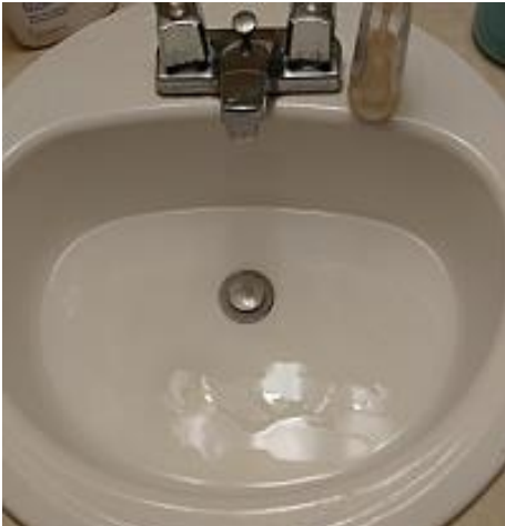
The sink drains slowly. Recommend Repair.
