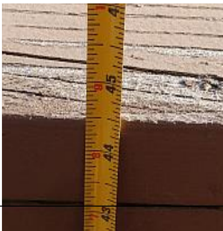
The railing is the proper height. Balusters are properly spaced.
