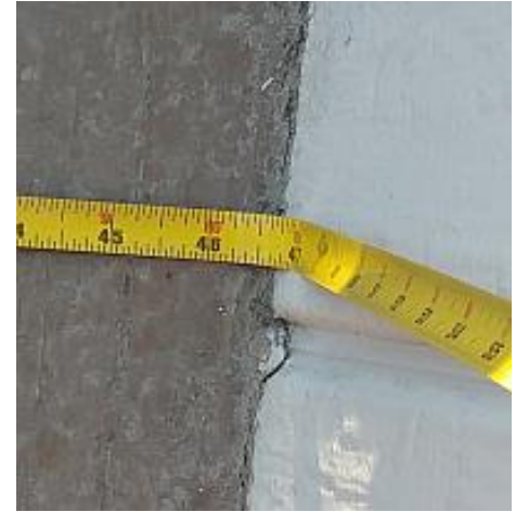
The floor is cantilevered 47 inches. According to current standards, cantilevers can extend up to one-fourth the back span of the joist. So the un-spliced joist would have to span 16 feet to allow the additional 47 inch cantilever. The joist structure is not visible so the inspector cannot make a determination if the cantilever is proper.
