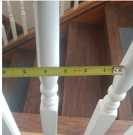
The stair guard is the proper height (36 inches minimum). Balusters are properly spaced (4 inches maximum).
