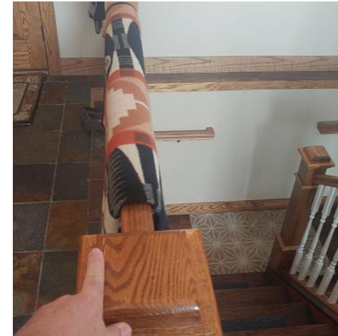
Loose stair guards observed. Recommend Repair.
