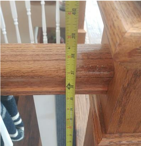
The stair guard is the proper height (36 inches minimum). Balusters are properly spaced (4 inches maximum).
